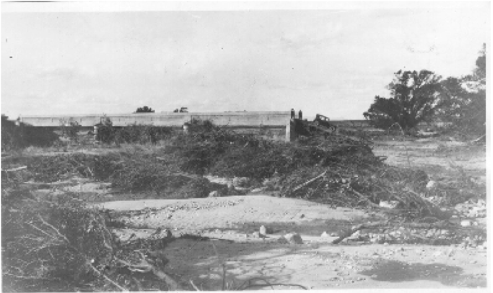
Historic Photograph Number fairbankbr-2 - no date given - Fairbank Bridge Upstream view, bridge showing drift and wash out of approach
